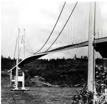
Figure 2.23 The Tacoma Narrows Bridge just before its collapse.
